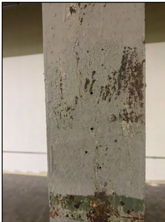
28: View of paint on vertical I-beams in low bay (PC-LB-3-1).
