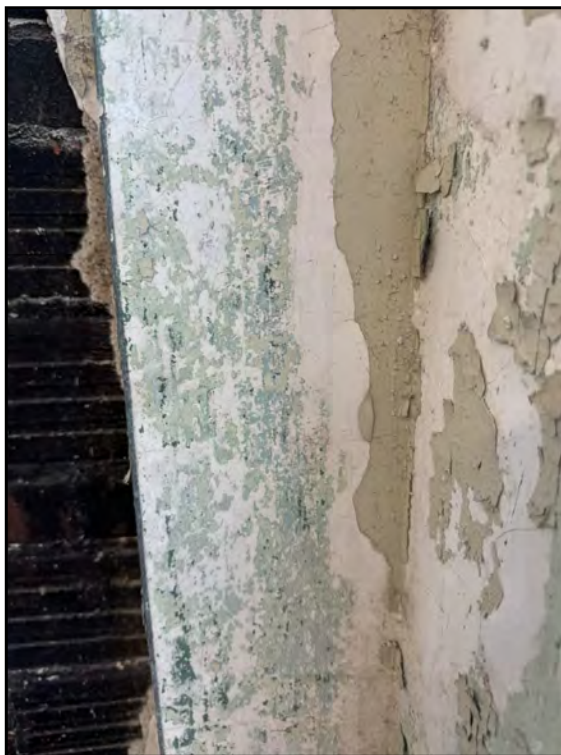
40: View of paint on plaster walls of the 6th floor office (PC-OF-7-1).
