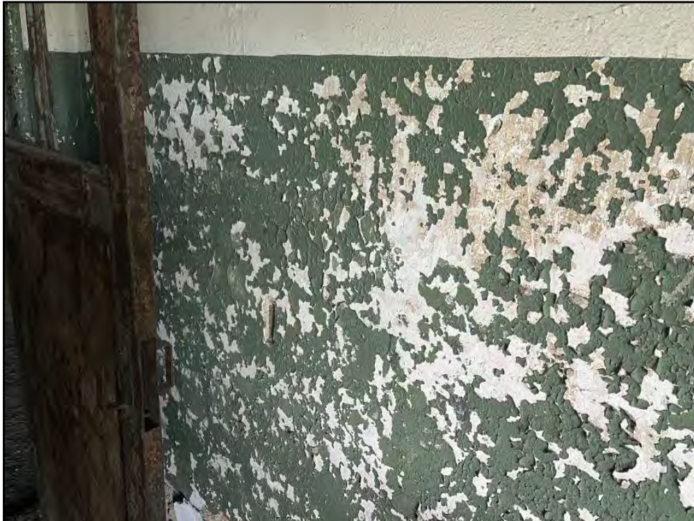
45: View of stairwell wall paint in north tower (PC-NT-8-2 and PC-NT-10-3).
