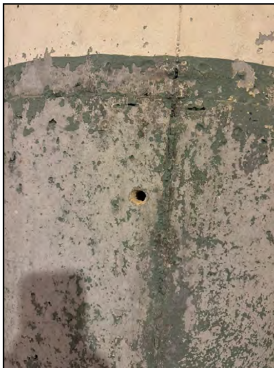
25: View of concrete pillar paint (PC-LB-1-1) and corresponding concrete sample (C-LB-1-1).
