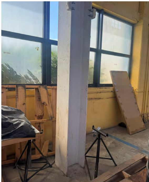
9. View of LBP on vertical metal beam in High Bay (#92)
