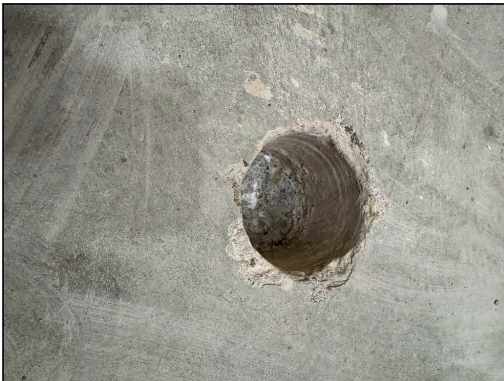
18: View of CF-OF-1 in 1st floor office area.
