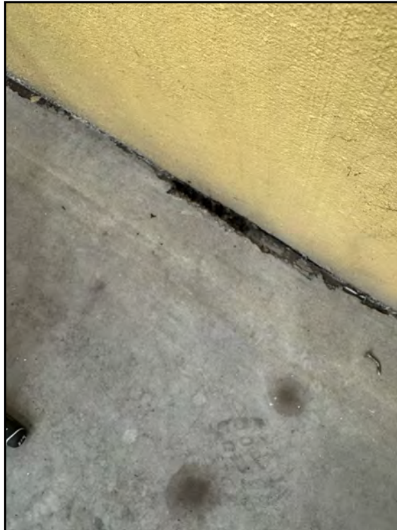
35: View of expansion joint along exterior walls of high bay (CK-HB-1-3).
