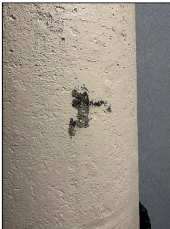
26: View of concrete pillar paint (PC-OF-1-3) collected from pillar on the 2nd floor.
