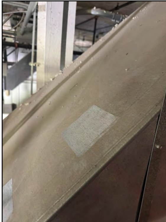
33: View of W-DS-6-2 wipe sample on ducts in diesel shop.
