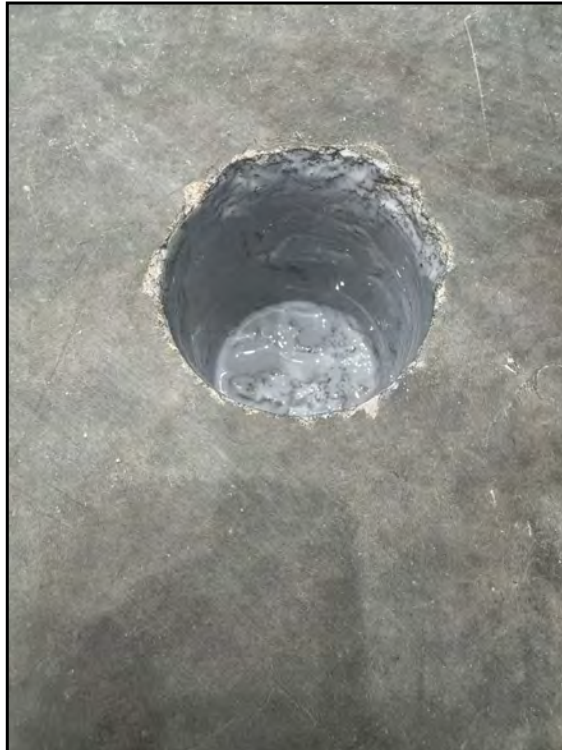
21: View of CF-SW-1 in high bay/south warehouse with epoxy seal.
