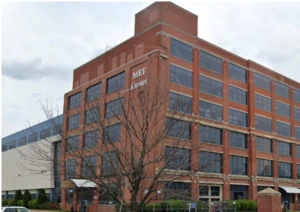
Representative view of south and west sides of the building.
