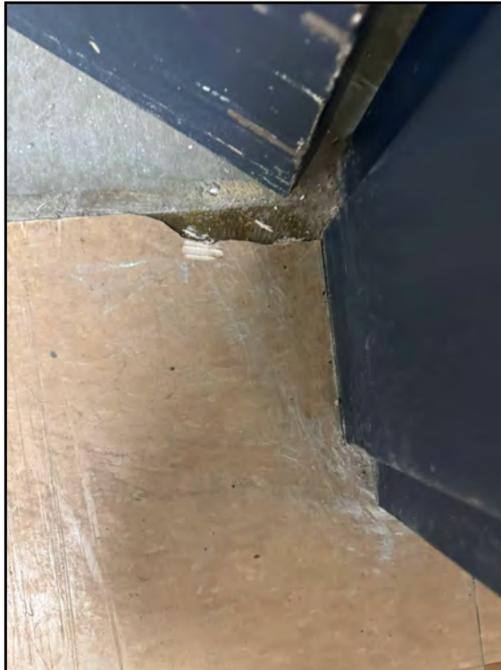
23: View of floor tile located in corridor between low and high bays (FT-LB-1-1).
