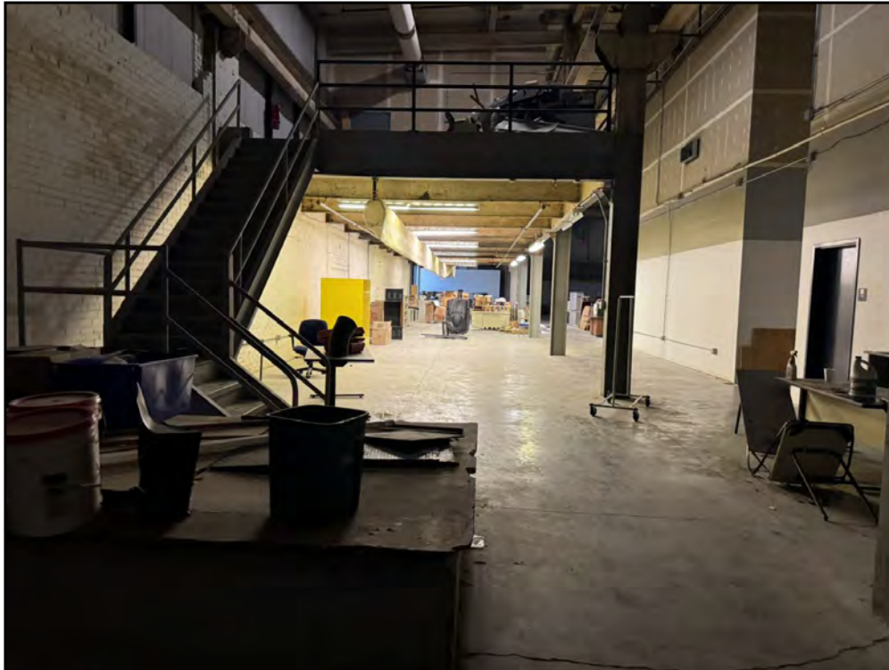
3: View looking towards the former Building 9A area and mezzanine in the low bay.
