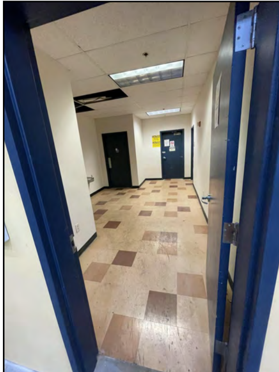
5: View of corridor between low and high bays.
