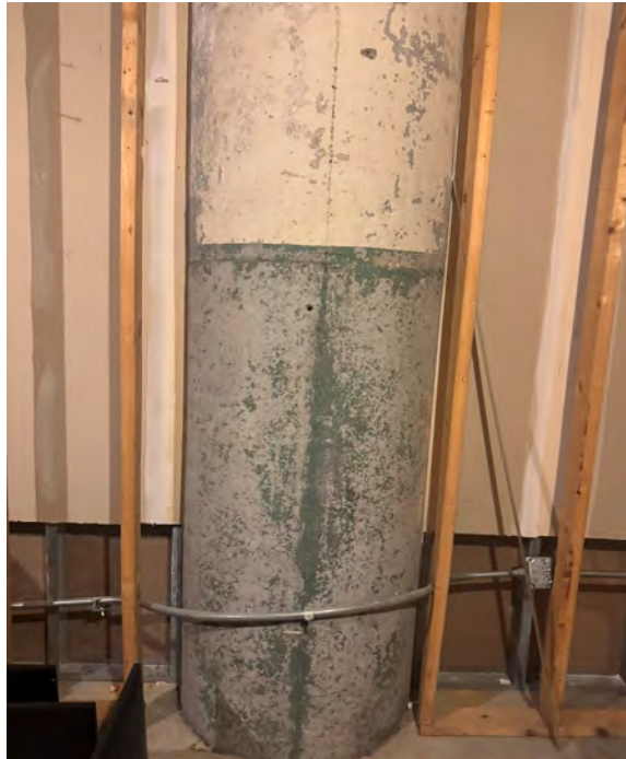
7. View of LBP on concrete pillar along south wall of Low Bay (#66, 67)
