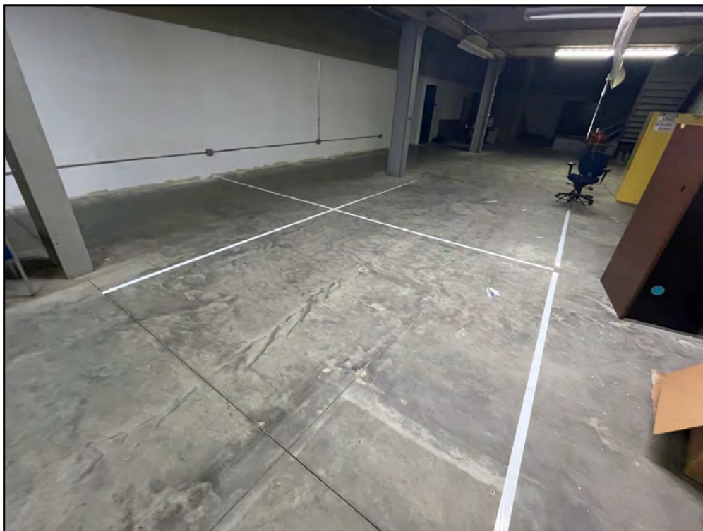
16: View of 10'x10' floor grid in the low bay/small transformer area.
