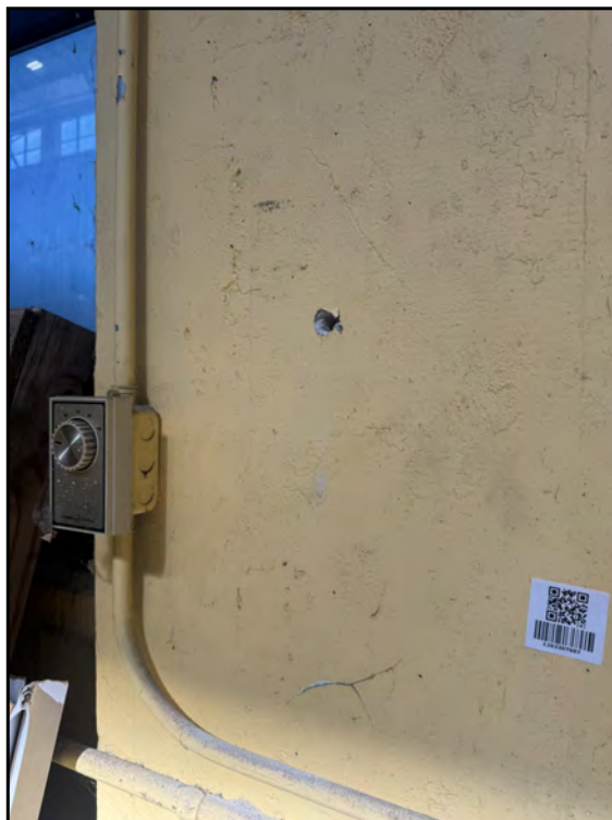
36: View of concrete column (C-HB-2-2) along west wall of high bay.
