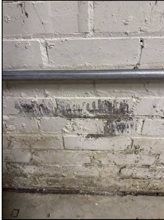
29: View of paint on east exterior brick wall in low bay (PC-LB-4-1).
