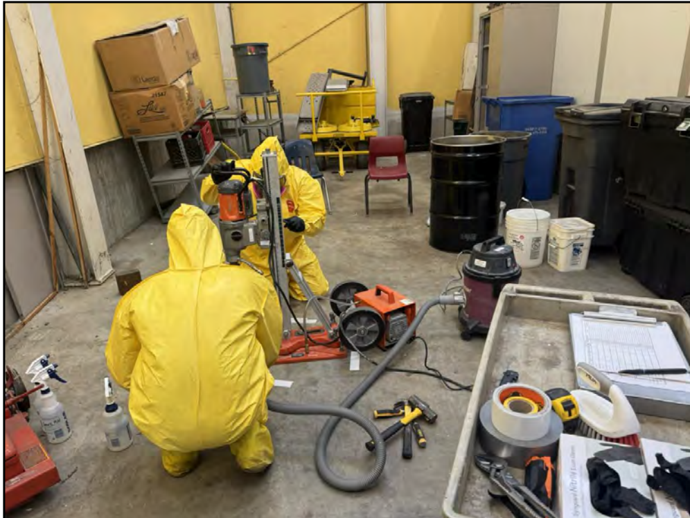
17: View of concrete coring activities in the high bay/large transformer area.
