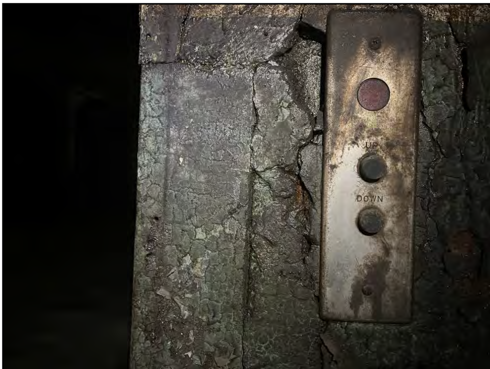
46: View of wipe sample area W-NT-12-1 on front of freight elevator on the 2nd floor of north tower.
