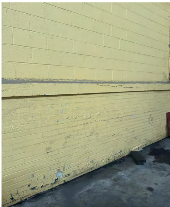
8. View of LBP on brick wall and concrete trim along northwestern side of High Bay (#79, 80, 81)
