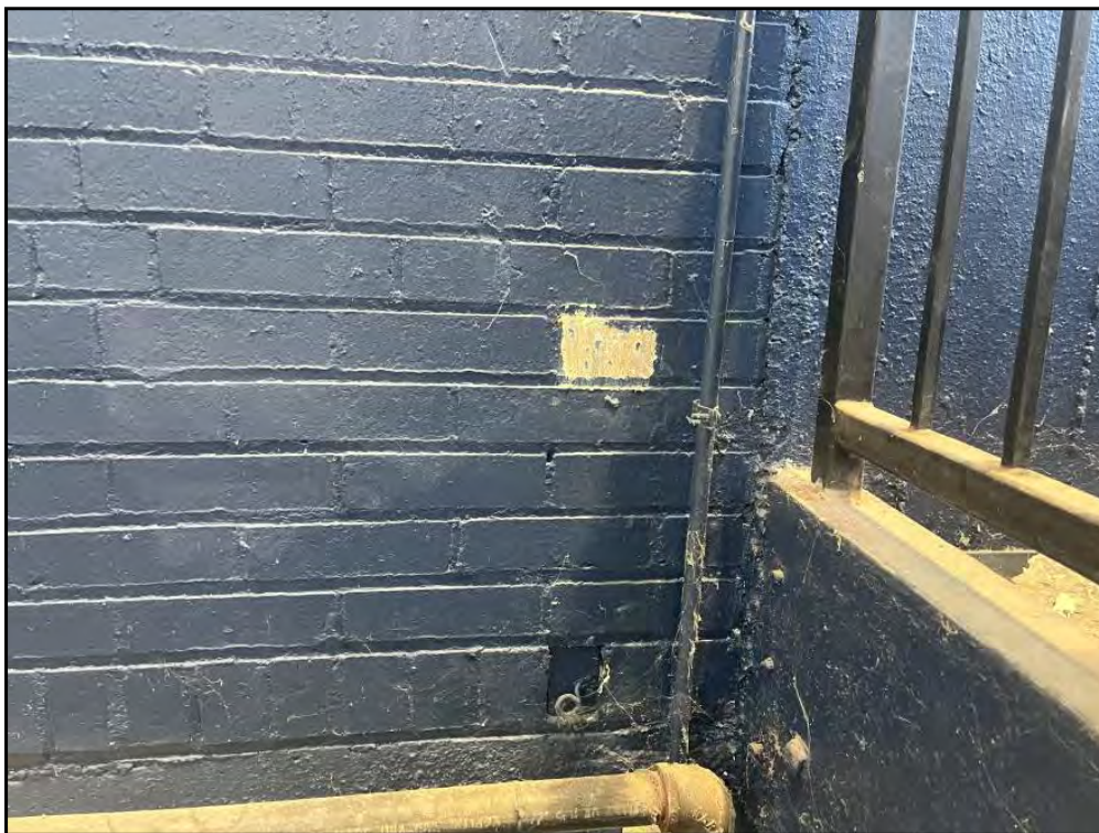
38: View of paint on brick wall on south wall of the high bay (PC-HB-6-3).
