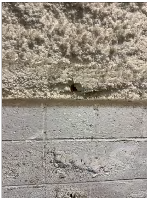
32: View of insulation in former window wells of diesel shop (I-DS-1-1).
