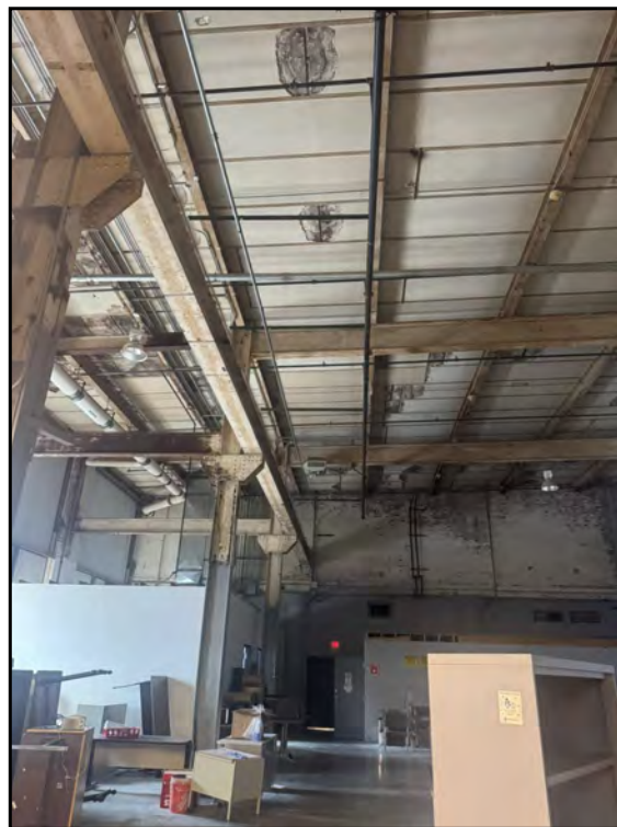
4: View of ceiling construction, cross beams and vertical I-beams in low bay.
