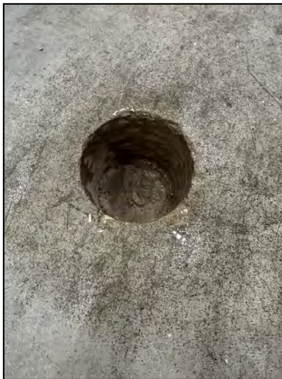
20: View of CF-LT-4 in the high bay/large transformer area.
