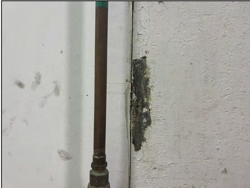
31: View of paint on vertical I-beams in diesel shop (PC-DS-3-3).
