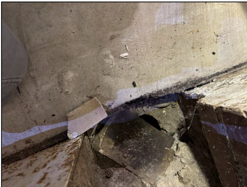
22: View of expansion joint along exterior walls of low bay (CK-LB-1-1).
